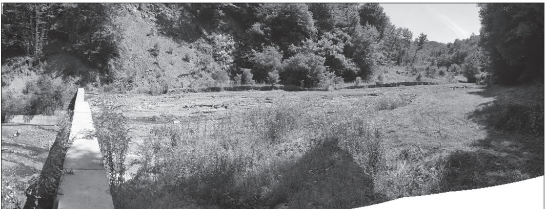
Figure 1. Check dam and aggradation on the Čađavica River, Jadar Basin, West Serbia
