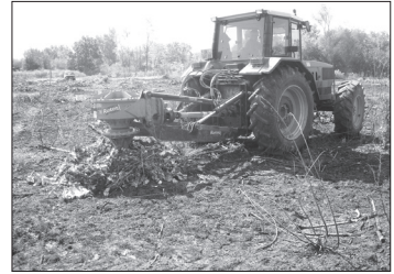
Picture 5. Stump chipping in SP3
