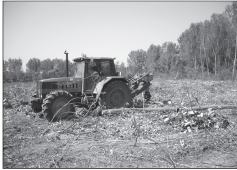
Picture 3. Stump chipping in SP1
