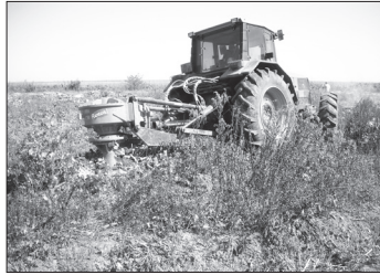
Picture 4. Stump chipping in SP2
